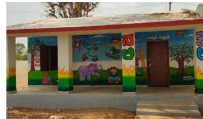
Inauguration of the newly renovated school in Kodagadala, India.
